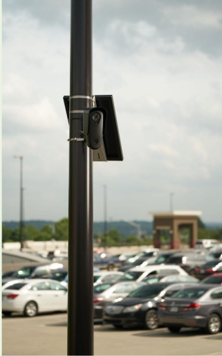
Solar & Existing Pole
