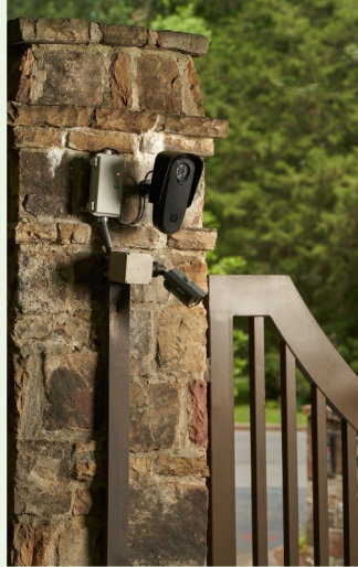
Electric & Existing Structure / Pole
